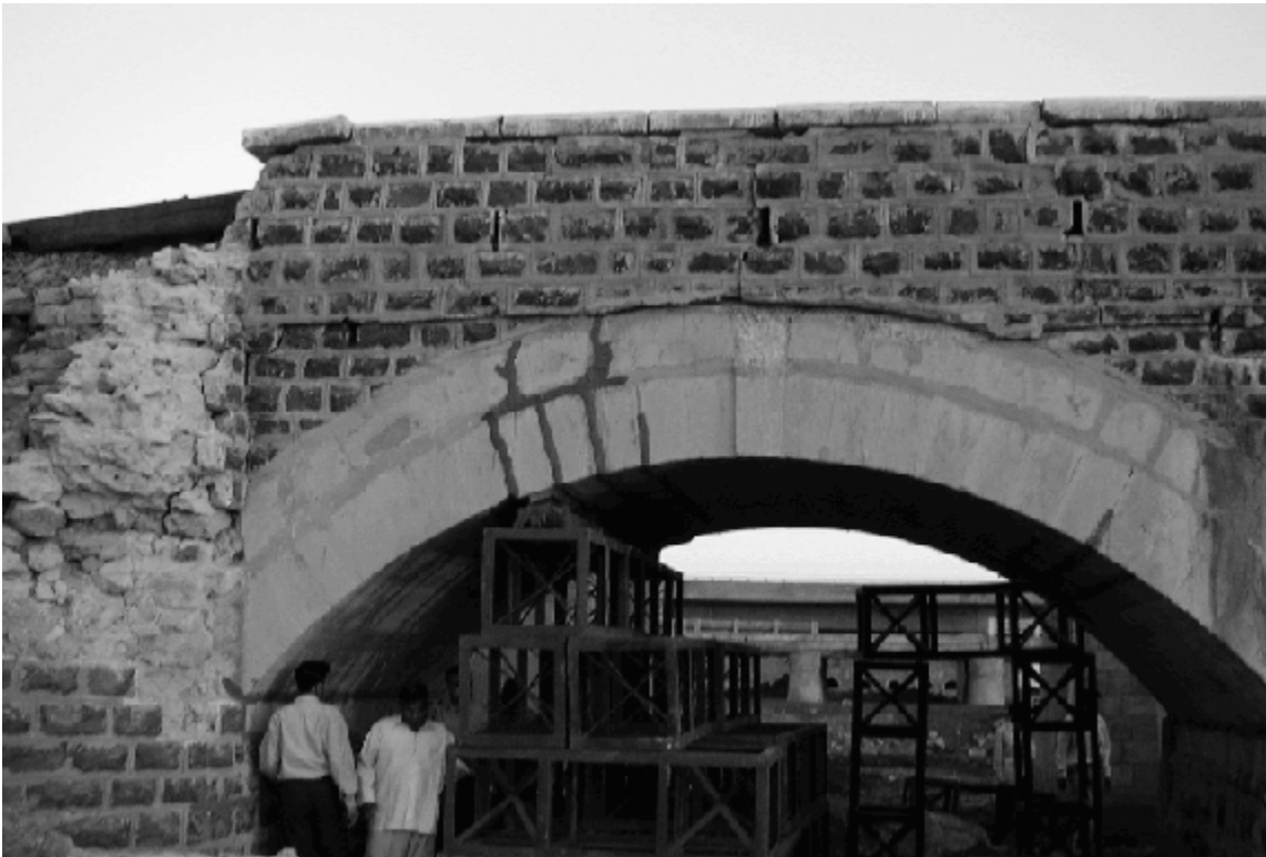
Figure 13. Epoxy injection repair of joints in arch ring at Bridge No. 261
