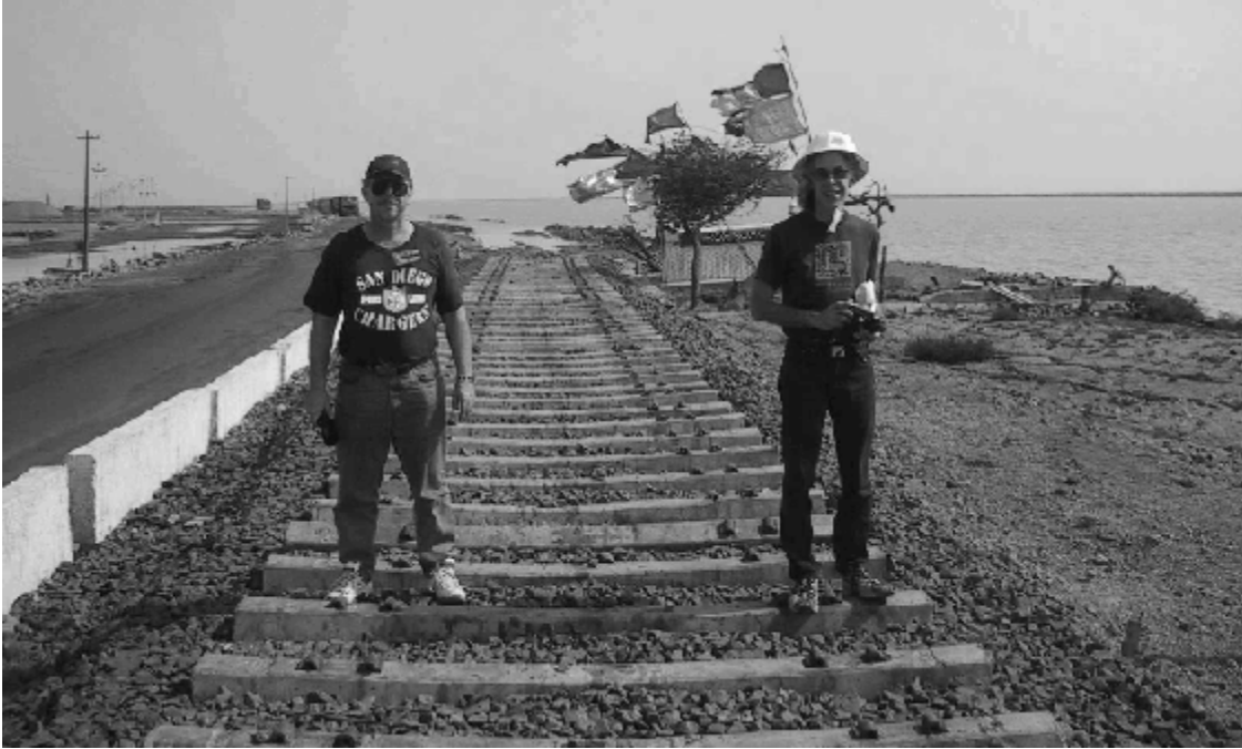
(a) Original alignment about March 1, 2001 (ASCE – TCLEE Earthquake Investigation Committee photo)
