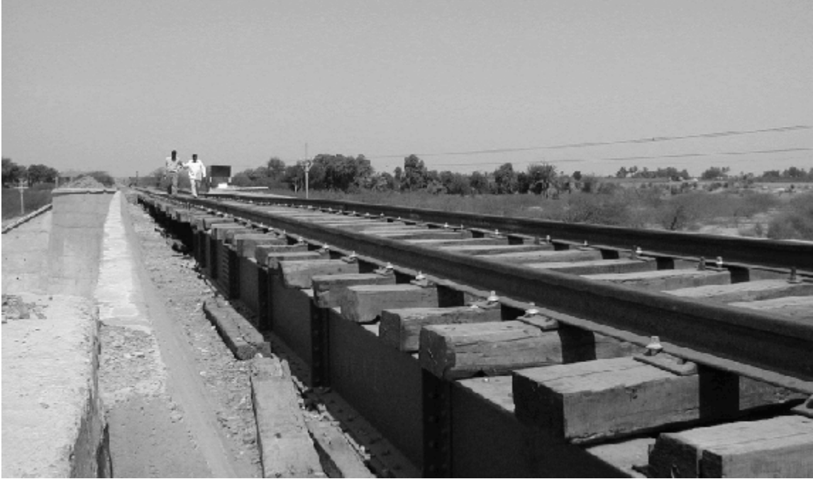
Figure 10. Falsework consisting of girders supported over piers at Bridge No. 48
