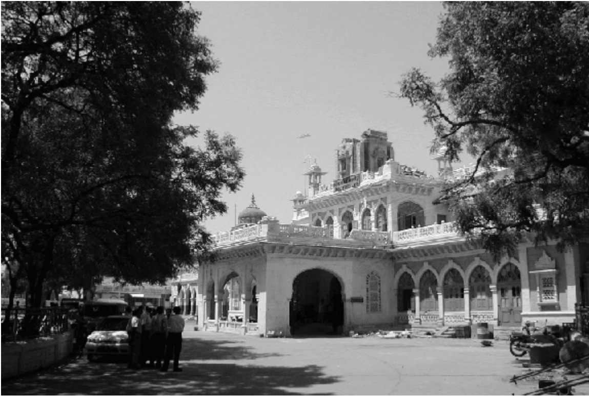
Figure 16. Morbi station after collapse of tower
