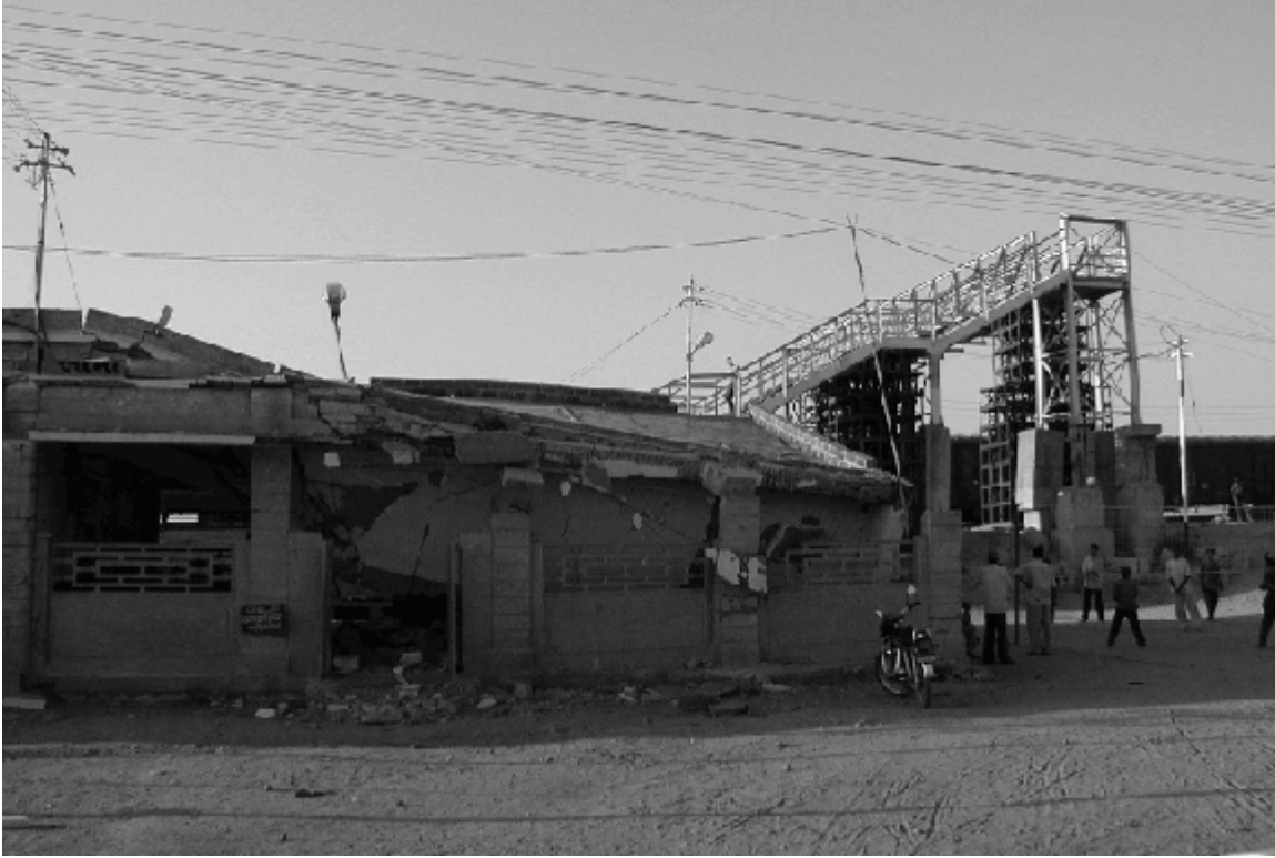
Figure 15. Samakhiyali station and foot bridge supported on cribbing
