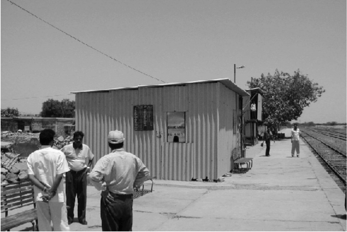
Figure 17 Temporary station and interlocking tower at Bhatiya
